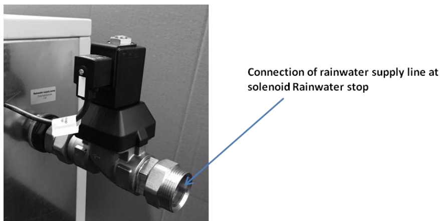
Figure 42: hydraulic connection of the Rainwater stop
