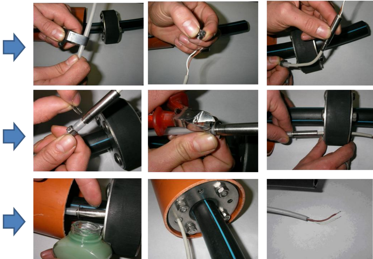
Figure 46: Installation of the connection cable with the stainless steel pipe
